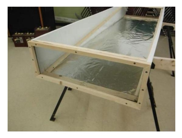
In this step, you'll be installing materials inside the collector box to absorb and transmit the sun's heat to the surrounding air. The "absorber" can be made of either charcoal-colored aluminum window screen or the type of metal lath used in plaster work. Although screen is easy to work with and relatively inexpensive, our tests found that lath produces higher temperatures. Because this design is for the *best* food dehydrator you can build, we recommend lath for the absorber material.
