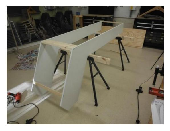
Before beginning assembly, you'll need to cut some braces to support the components of the solar dehydrator on the interior. Most of these braces will serve more than one function so it's important to use the correct one at each location. See the detailed drawing ("How it Works," above) for proper sizing and placement of the braces.
