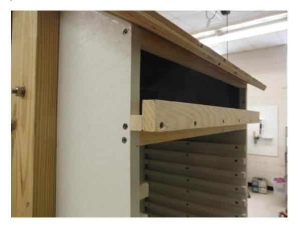
To install the back vent covers, you'll first need to build up the 1-1/2-inch-wide brace at this location so it can support both the covers and the door (which you'll install next). Attach a 3/4-by-3/4-by-24-inch strip of wood to the top half of the brace, and then screw a 1-1/2-by-3/4-by-24-inch wooden piece to the top of the strip you just placed on the brace. Drill pilot holes to avoid cracking the wood, and be sure to stagger the screws for the first and second strips.
